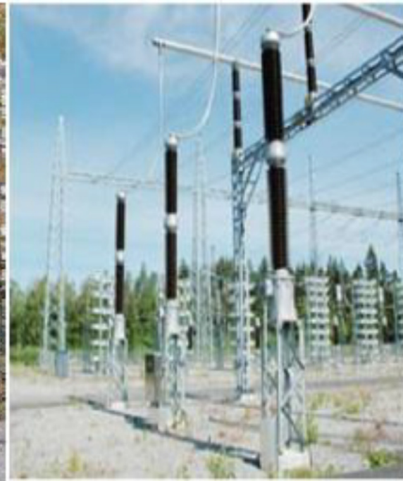
Figure 19-Inductive voltage transformer
