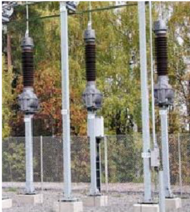
Figure 19-Inductive voltage transformer
